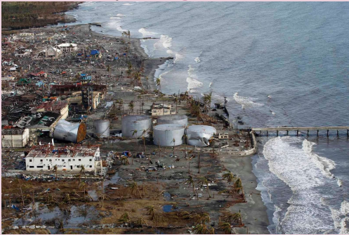
Damaged fuel tanks on the Tanawan coast. (Source: AP Photo/Wally Santana )
